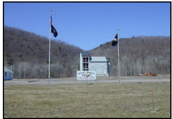
Figure 15. Richard L. Hanson Fire Training Center in Yosts
